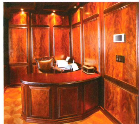
Veneers are used to give an attractive finish
