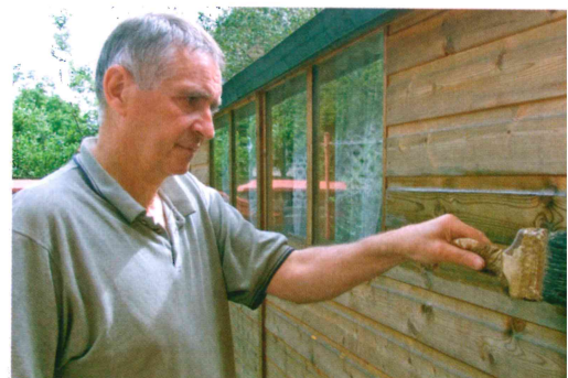
Applying preservative – protective gloves and glasses should be worn
