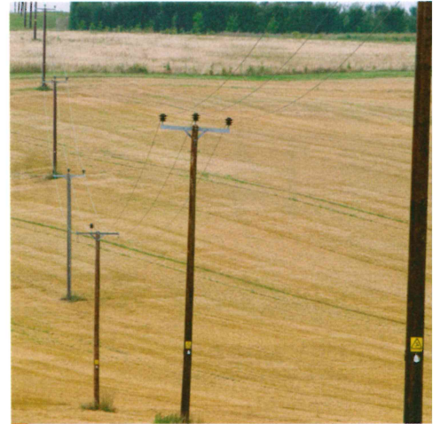
Telegraph poles have to be treated with oil preservative to ensure long life
